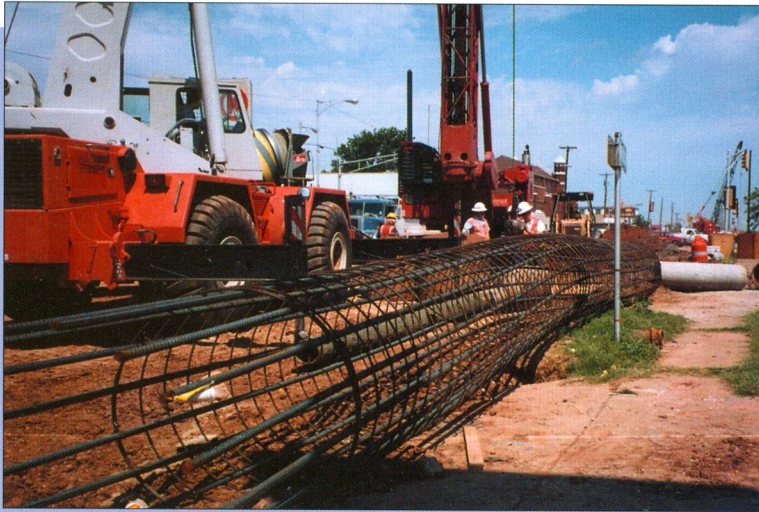
Full length reinforcing cages for all shafts.
