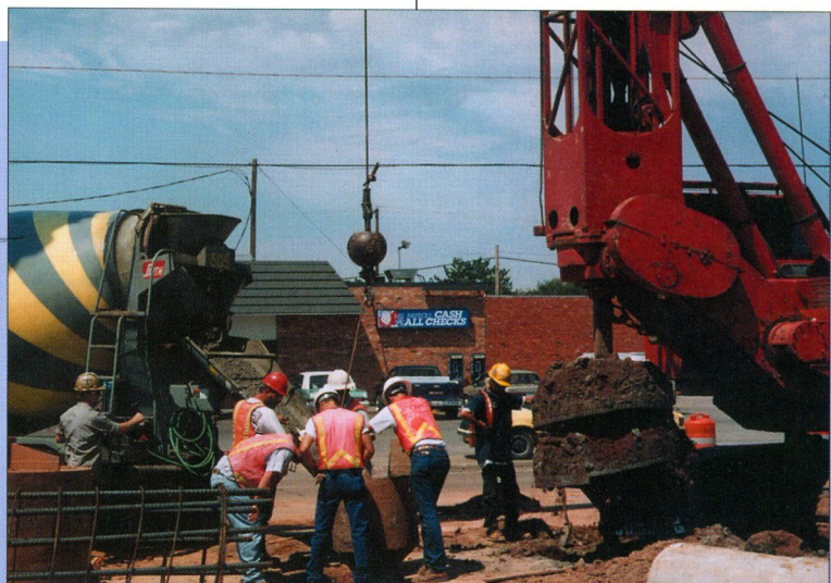
Material on auger confirms expected soil profile.
