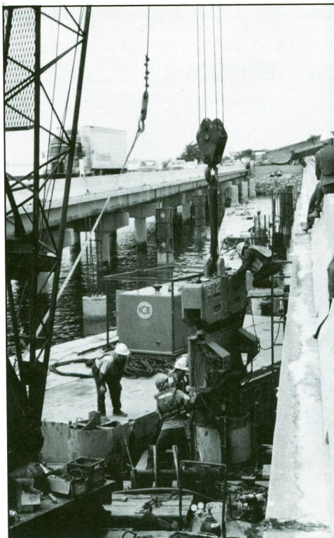
Vibrating casing (left) and placing reinforcing cage (right) under very tight working conditions. Drilled shafts and bridge piers in various forms of completion are visible.
