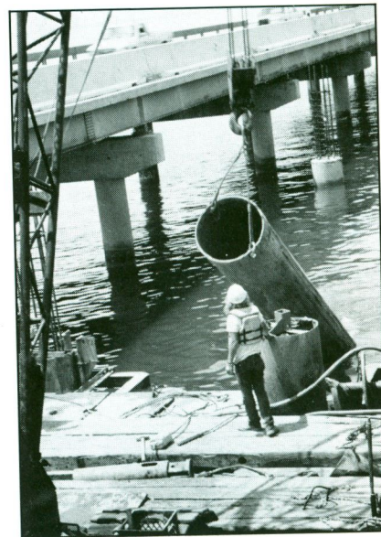
Casing on its way to lake bottom storage. Finished drilled shaft (center right) with extended reinforcing.
