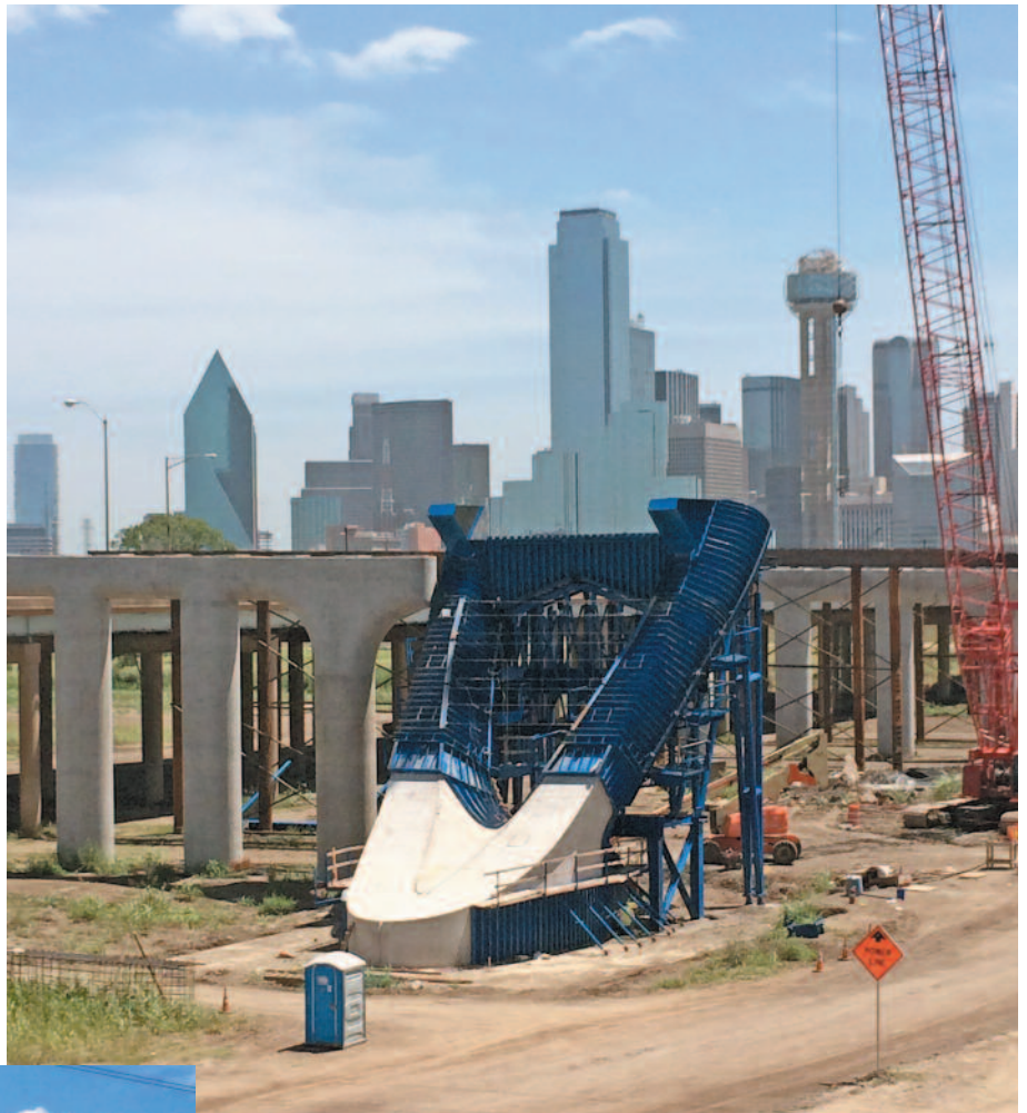
Architectural column being formed.
