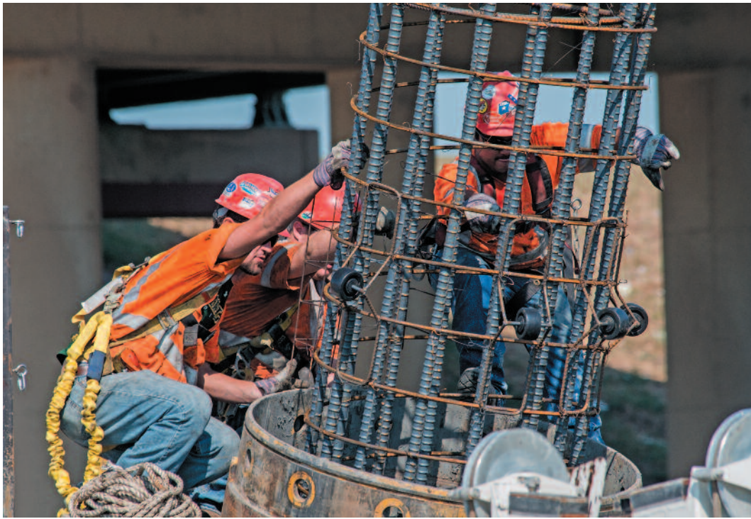
Critical rebar placement.
